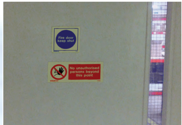
8064PT (No unauthorised persons beyond this point) & 5421C (Fire door keep shut)
